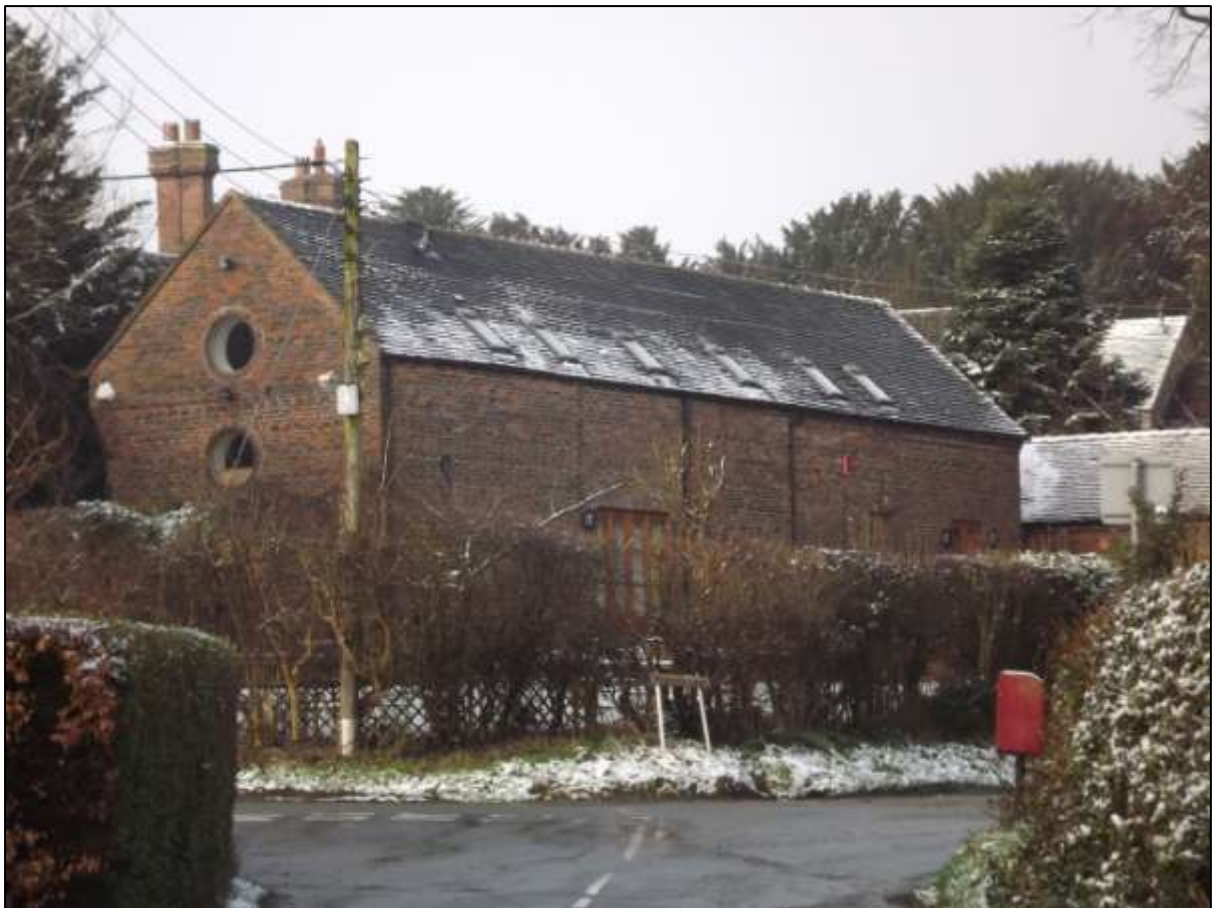
Figure 6 Grade II listed, 18th century Village Farm Barn
