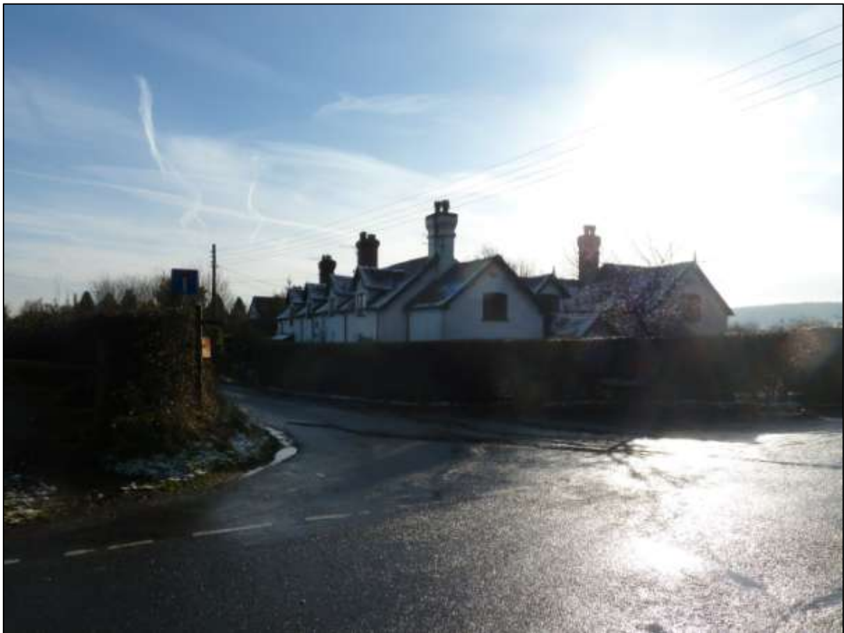
Figure 20 The crossroads at Hanchurch Lane facing south towards Ridding Bank
